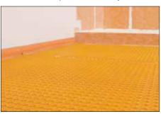
4 Abut end and side sections of adjacent sheets. **Note:**Aligning the studs on the top of the matting during installation can help make subsequent heating cable installation easier.
