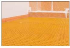
Abut adjacent sheets and align the studs on the top of the matting to make subsequent heating cable installation easier.
