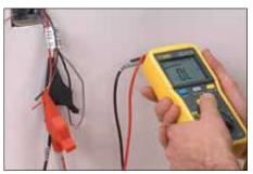
Once the tile installation is complete, retest the heating cable and record values in the heating cable tests log (page 39).
