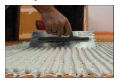
Tile can be installed over DITRA-HEAT and DITRA-HEAT-DUO immediately; no need to wait for the mortar to cure. Fill the matting with SET, ALL-SET, FAST-SET, or unmodified thin-set mortar and comb additional mortar over the matting using a trowel that is appropriate for the size of the tile.
