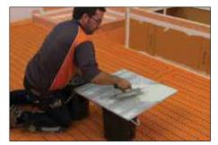
Periodically remove and check a tile to ensure that full coverage is being attained.
