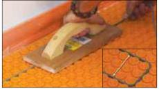
4 Embed the heating cables between studs utilizing the recommended pattern, at a spacing determined in the **Spacing Details** section on page 20-21.
