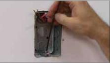
Thread the heating cable cold lead through a conduit from the base of the wall to the thermostat electrical box. Floor temperature sensors need to be threaded through the same conduit containing the cold lead, or within a separate conduit.
