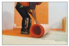
Apply DITRA-HEAT or DITRA-HEAT-DUO to the floor, fleece side down. Solidly embed the matting into the mortar using a float, screed trowel, or DITRA-ROLLER, making sure to observe the open time of the bonding mortar. If the mortar skins over prior to matting installation, remove and reapply. **Note:** It may be helpful to back roll the DITRA-HEAT matting before installation to help the membrane to lay flat.
