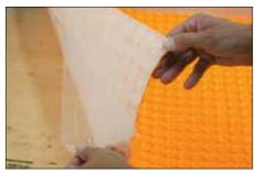
Remove release liner from DITRA-HEAT-PS / DITRA-HEAT-DUO-PS membrane.
