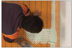
Comb additional SET, ALL-SET, FAST-SET, or unmodified thin-set mortar over the joint using a 1/4" x 3/16" (6 mm x 5 mm) V-notched trowel or the KERDI-TROWEL, which features a 1/8" x 1/8" (3 mm x 3 mm) square-notched design.
