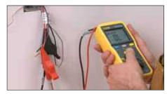
Once the heating cable and floor temperature sensor installation is complete, retest and record values in the heating cable tests log (page 39).
