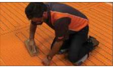
Use care not to damage the cables during installation, particularly before the cables are embedded in the matting
