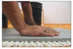
Solidly embed the tiles in the setting material, sliding the tile back and forth perpendicular to the tile ridges underneath. This will help collapse the mortar ridges and improve contact between the mortar and the tile. Make sure to observe the open time of the bonding mortar. If the mortar skins over prior to tile installation, remove and reapply.
