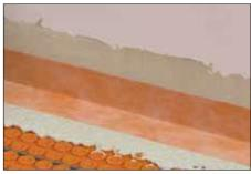
4 all wall junctions, apply KERDI-BAND as described in steps 1-3, centered where the wall and floor meet. In some applications the vertical section of the floor/wall transition will not accept a bond to unmodified thin-set mortar. Connections to such elements can be achieved using KERDI-FIX sealant and bonding compound or suitable trowel-applied waterproofing materials, such as those that require atmospheric moisture to cure (e.g., urethane sealant).
