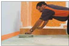
Using a thin-set mortar that is suitable for the substrate, apply the thin-set mortar (mixed to a fairly fluid consistency, but still able to hold a notch) using the DITRA-HEAT trowel, or other 1/4" x 1/4" (6 mm x 6 mm) square-notched trowel.
