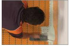
1 At the joints, fill the matting with SET, ALL-SET, FAST-SET, or unmodified thin-set mortar, approximately 8" (203 mm) wide, centered over the joint.
