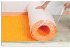
2 Apply peel-and-stick membrane to the floor, fleece/ adhesive side down. Solidly embed the matting into the substrate using a float, screed trowel, or DITRA-ROLLER. Proper installation results in full contact between the adhesive and substrate beneath.
