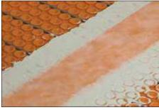
Apply 5" (127 mm)-wide KERDI-BAND, centered over the joint. Using the flat side of the trowel, firmly press the banding into the mortar to ensure 100% coverage and to remove excess mortar and air pockets.
